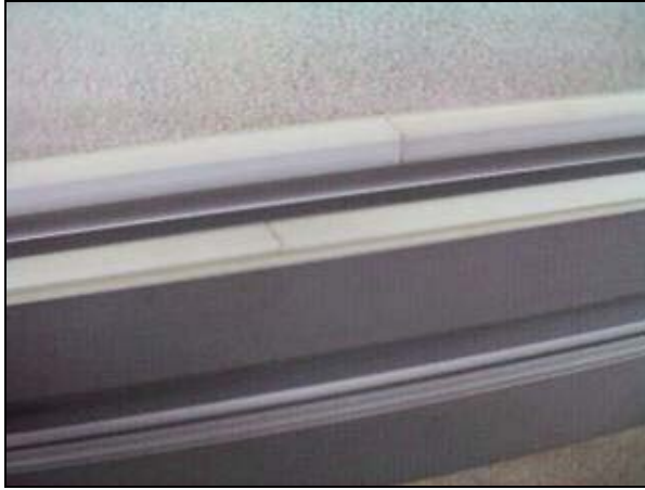
Mount the sliding grib in an offset way
