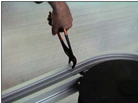
Check the butt joints and transitions
